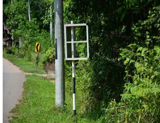
Gambar 2.27 Chevron Delineator Hilang
